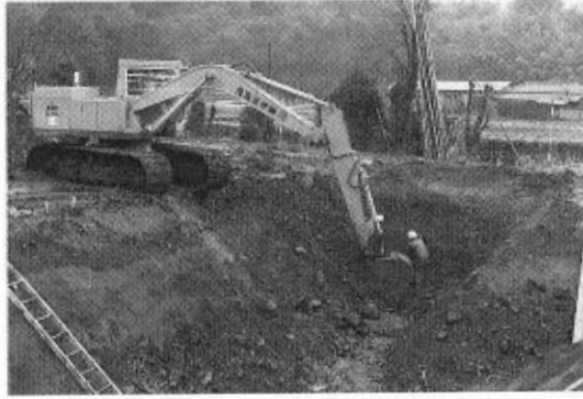
Fig. 3. Trench opening work at Ukihashi.
