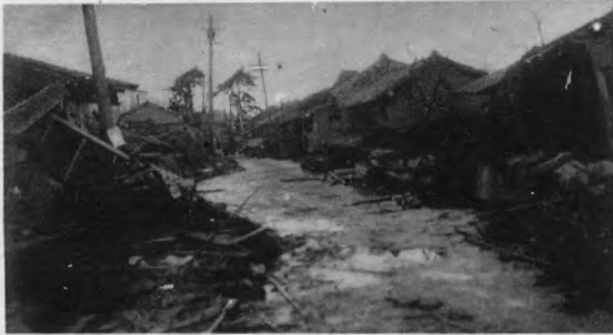
Fig. 3. Wrecked Houses in Iwataki-machi.
