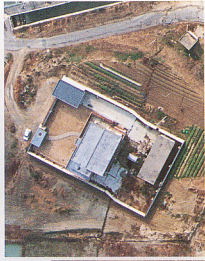
Dislocated house by the earthquake fault (Awaji Island) (by Asia Air Survey)
