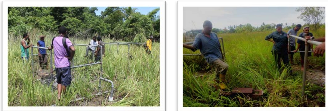
Figure 4 – Vandalized solar operated water supply system.
