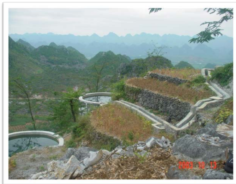
Fig. 1. Water Storage Project for Epikarst Springs in Guohua Town, Pingguo County, Guangxi-Solution to the Engineering Water Shortage
