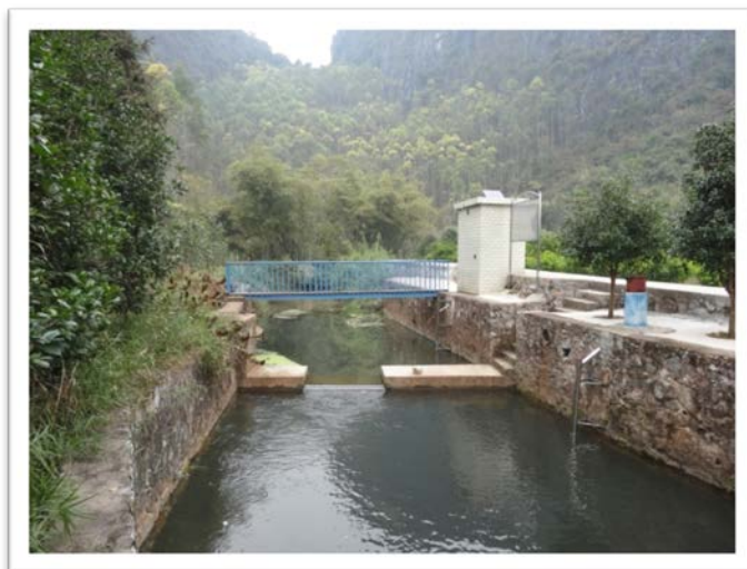
Fig. 8. Groundwater Flow Rate Monitoring through Multilevel Rectangular Weir in Subtropical Monsoon Climate Area---Zhaidi Underground River, Guangxi
