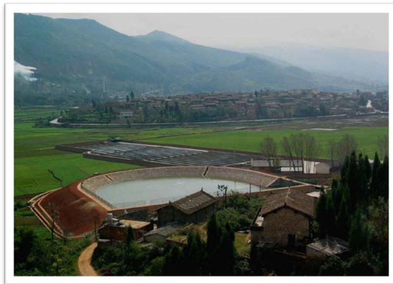
Fig. 7. Restricting Flow Rate and Adjusting the Pressure by Damming Large Karst Springs in Pijiazhai, Luxi Basin
