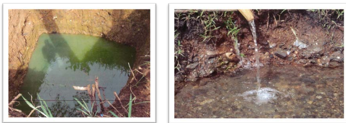
Figure 2 – Top: Moderately consolidated hill-slope deposit in exposed excavated pit toilet. Right: Trench dug by a staff member, in the swampy area opposite the school for water supply.
