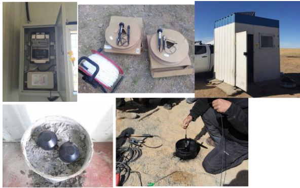
Photo 2 Groundwater monitoring (installation)
