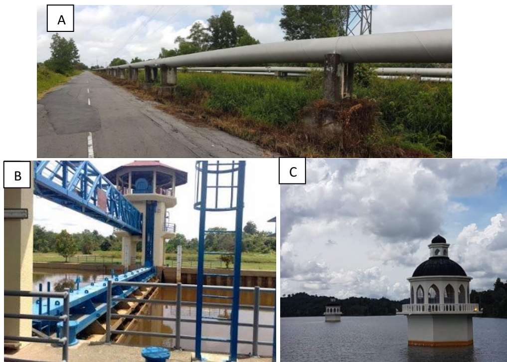
Fig. 3. (A) Badas pumping station, (B) Benutan dam and (C) Mengkubau dam
