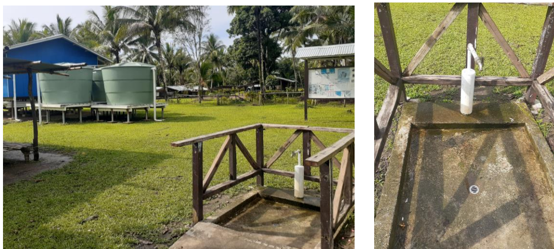
Fig. 6. Rainwater catchment tanks connected to tap outlets in a village in Western Province.
