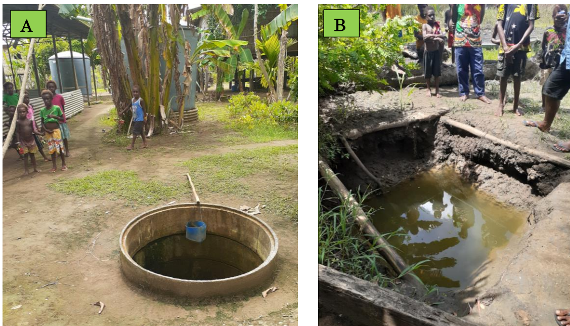
Fig. 5. Shallow wells, lined (A) and unlined (B) that experience saltwater intrusion due to close proximity to the coastline; South Fly District, Western Province.
