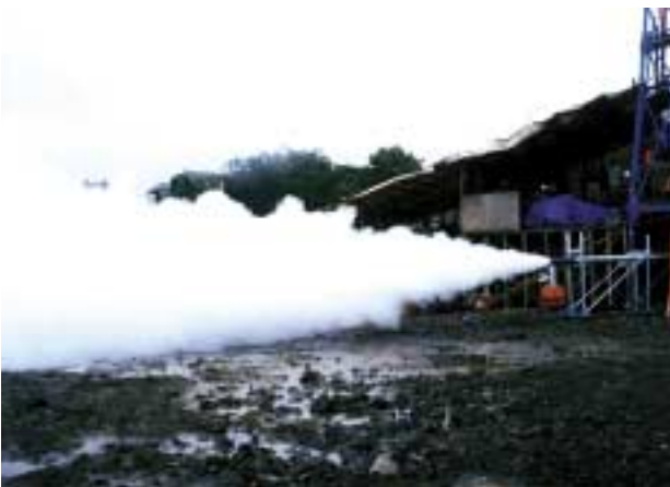
Fig.15 Photograph of the flow test of NEDO MT-2 well. It was successful. About 15 tons per hour of dry steam were stably produced at an entirely valve open state. Considering the shallower well depth of 162.35 m, the production rate is quite economical.
