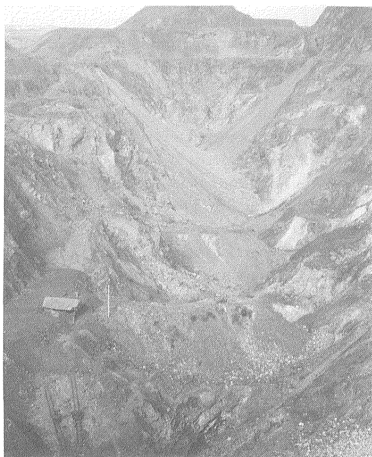
Fig. 7 Open pit part of the Fenghuagshan iron deposits. The left half is the sedimentary wall rocks including the orebody dipping about 45^\circ to the left, and the right half is the intrusive subvolcanic rocks.
