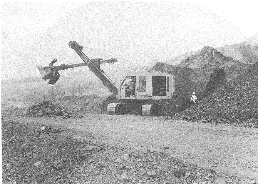
Plate 10-2 Workings of raw material shale of Bilton.
